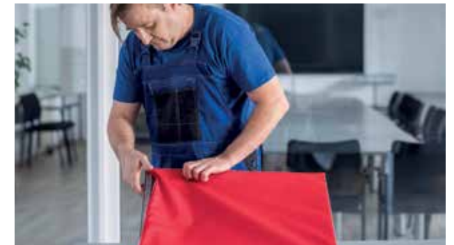
Fit the other flow panel on a plenum box
