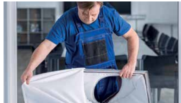
Peel off the flow panel
