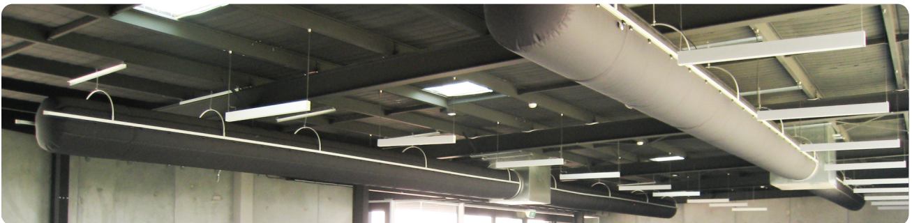
Fabric-based air distribution delivers uniform, low-velocity supply air across an entire space – controlled and measurable, regardless of season.
