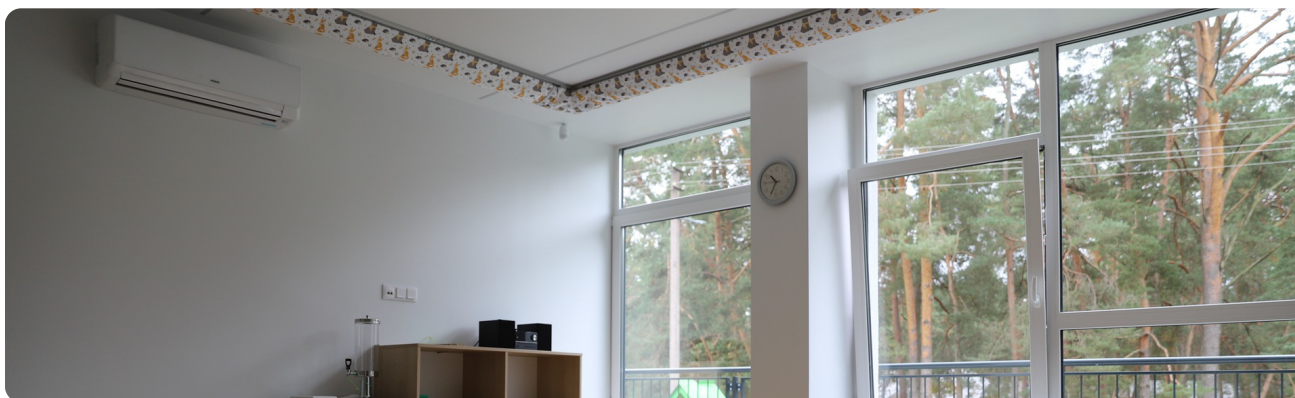
Lightweight, machine-washable fabric ducts integrate easily into both new and existing school buildings.
